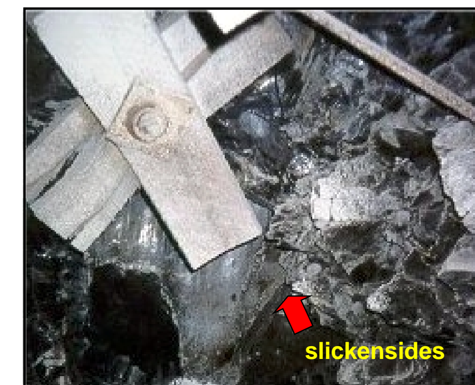
Figure 10. Slickensides at different orientations in fireclay exposed in the roof above the Baker coal bed after a fall.
