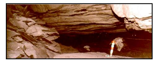
Figure 17. Stackrock strata in roof fall above Lower Elkhorn coal
