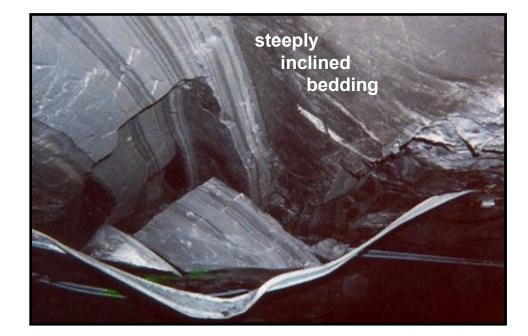
Figure 14. Roof fall exposes steeply dipping beds
