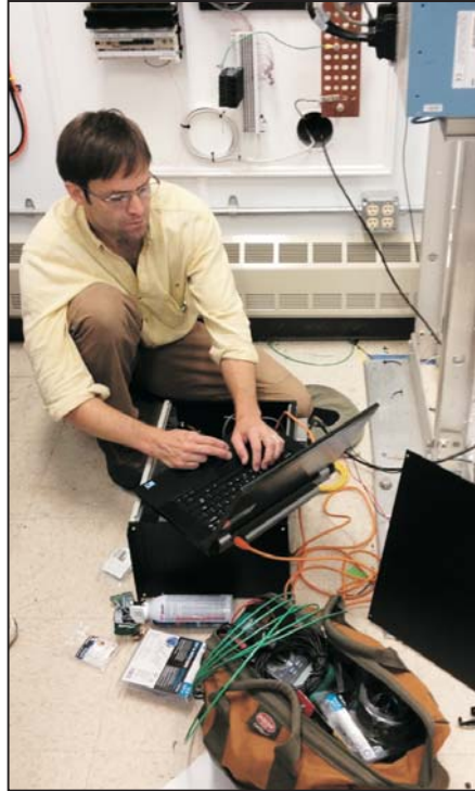
Seth Carpenter installs and tests a new seismic instrument at station SMKY in the Kentucky Emergency Warning building near Sacramento. He upgraded the analog station with digital equipment.
