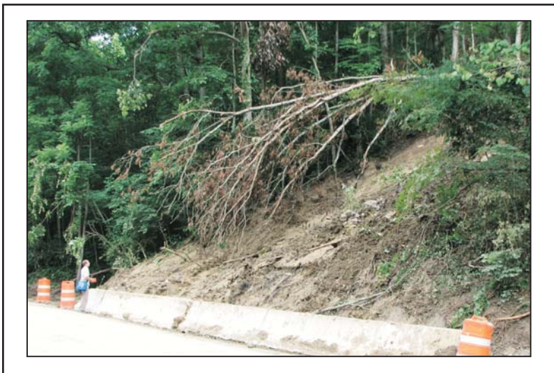
As part of his landslide inventory, Matt Crawford has visited multiple sites to gather information on slides and damages.
