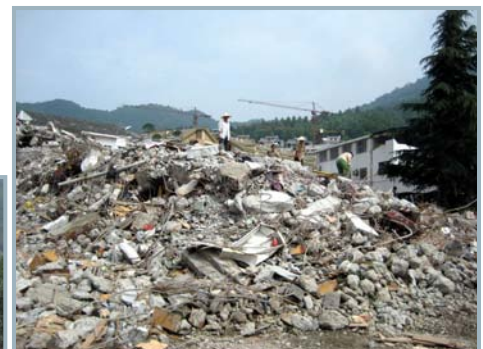
People pick through the pile of concrete that remains from a building which completely collapsed.
