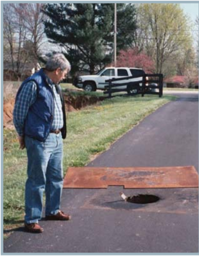
A property owner in Franklin County looks at the damage to his driveway from a cover-collapse sinkhole which staff in the Water Resources Section investigated in April 2008.
