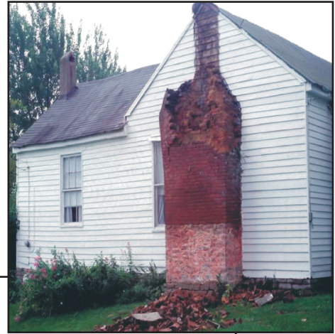
Figure 5. (a) Damage to a home in Maysville caused by amplified ground motion (shaking) from the 1980 Sharpsburg earthquake. (b) Building collapse caused by strong ground motion of the 2008 Wenchuan, China, earthquake (magnitude 7.9).
