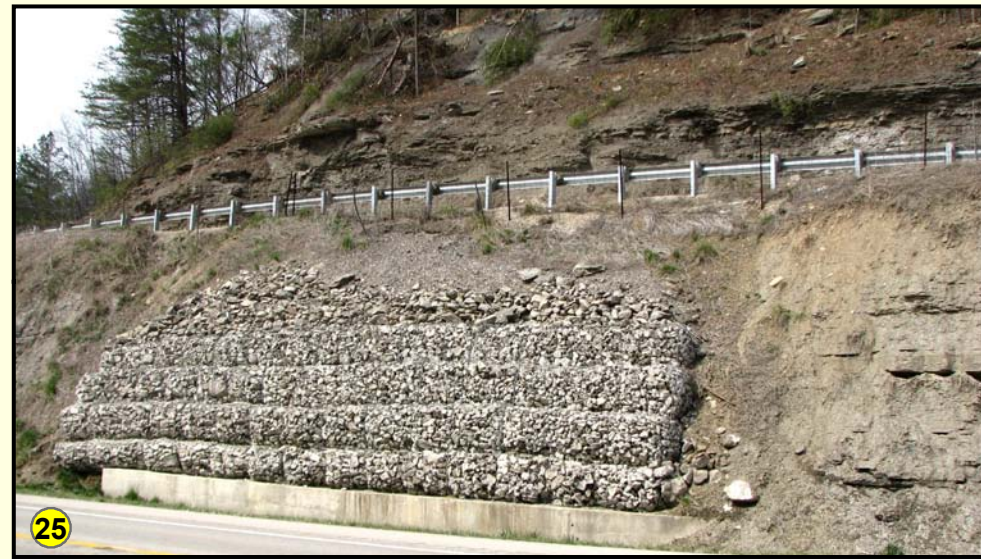
Mile 63.6: Roadcuts into shale of the Hyden Formation (Ph) may require support for stability.
