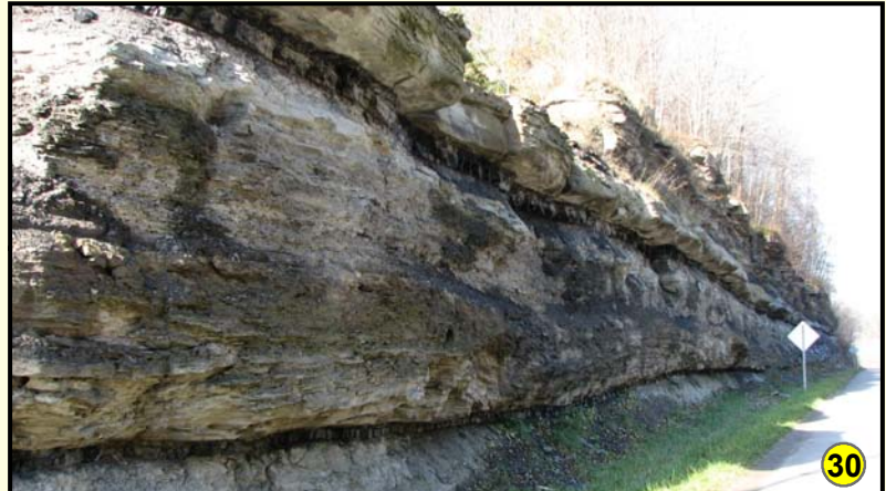
Mile 1.8: Fire Clay coal (fc) above an unnamed coal bed in the Hyden Formation (Ph).
