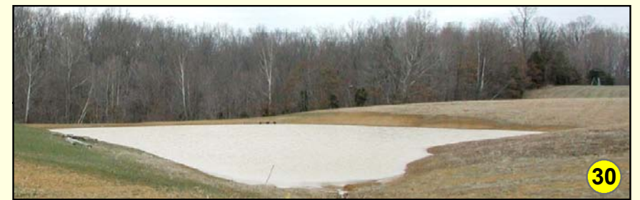
Most ponds constructed on shale units, such as this one off of Ky. 2766 just south of the parkway, are successful.
