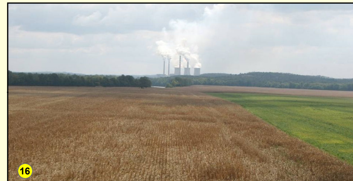
Mile 65.6: The Tennessee Valley Authority Paradise coal-fired power plant is located on the Green River near the village of Paradise. The plant has three units, completed between 1963 and 1970, and three large natural-draft cooling towers to provide cooling water. In 1985, a barge unloading facility was added so that coal could be delivered by barge as well as by rail and truck.
