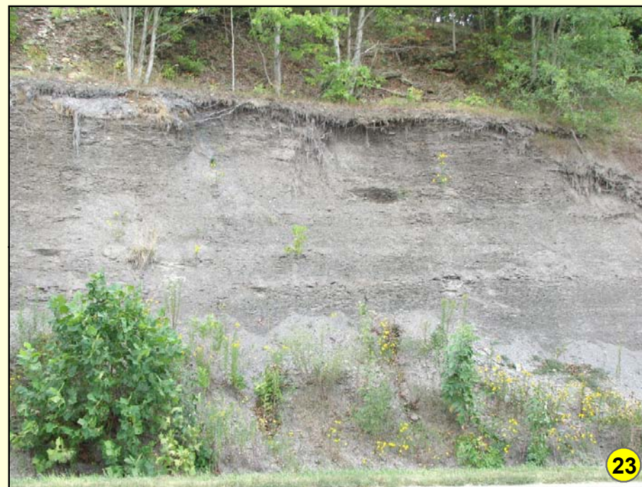
Mile 91.6: Shale unit of the Tradewater and Caseyville Formations (Ptc). When exposed to air and water, shale breaks down quickly. It is unstable on slopes, makes a poor foundation, and requires drainage management. It does provide an impermeable seal for ponds and waste-disposal areas.
