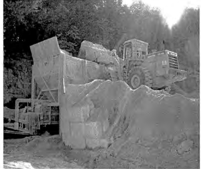
Figure 35. Dense grade or crushed stone base added to pug mill.
