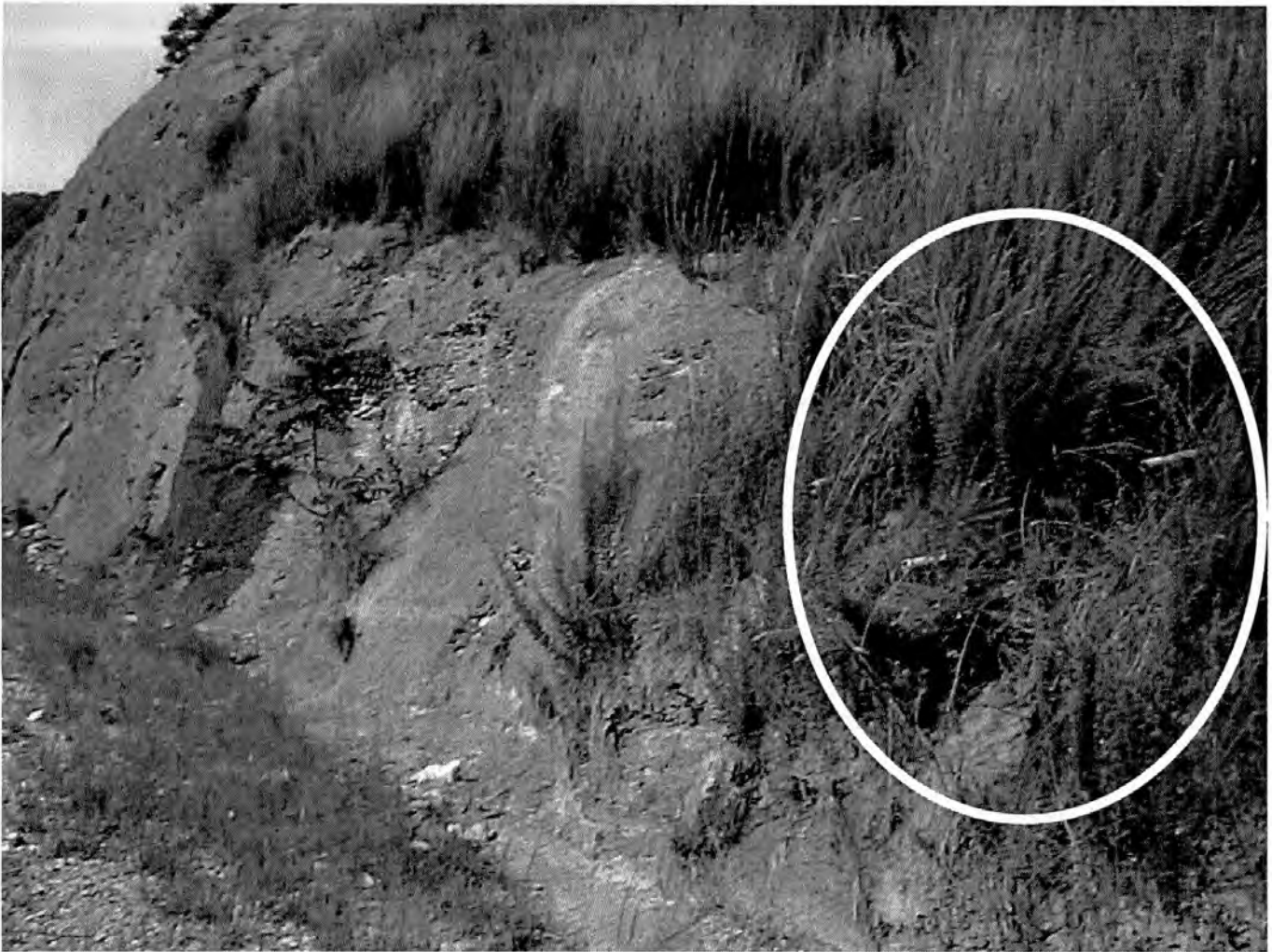
Figure 10. Completed project with three drainage pipes (right side in grass) in the Borden Formation.
