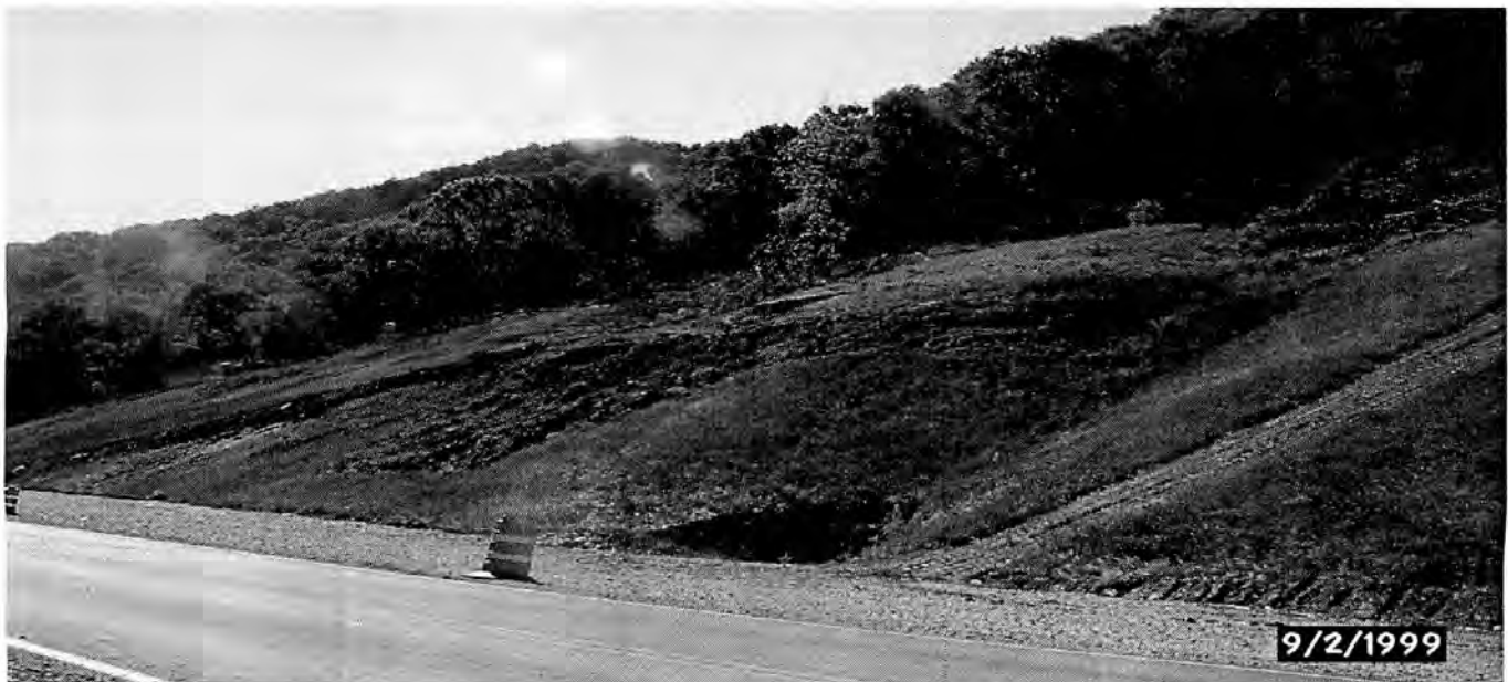
Figure 7. Failed slope during construction of Ky. 421.
