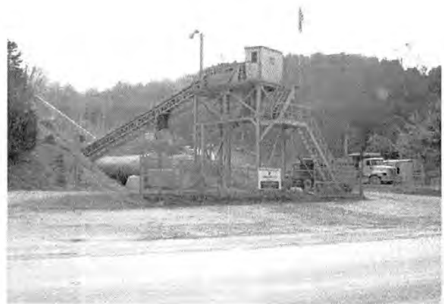
Figure 36. Water mixed with crushed stone to be used on roadway.
