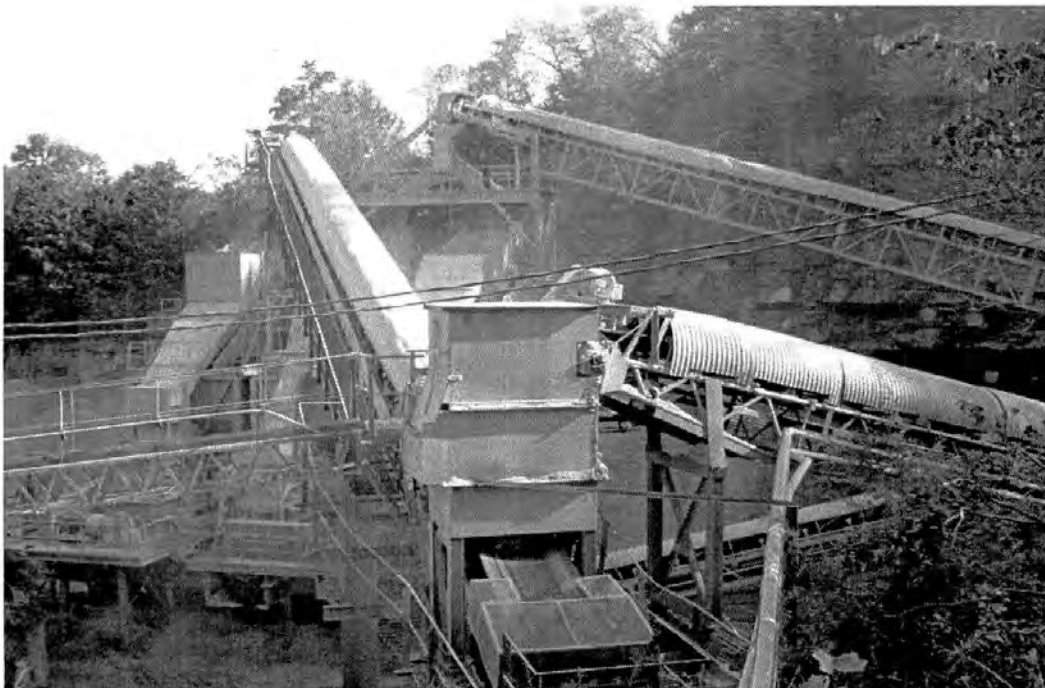
Figure 32. Conveyor belt system.
