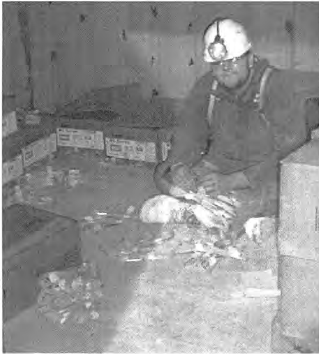
Figure 29. Explosives being prepared.
