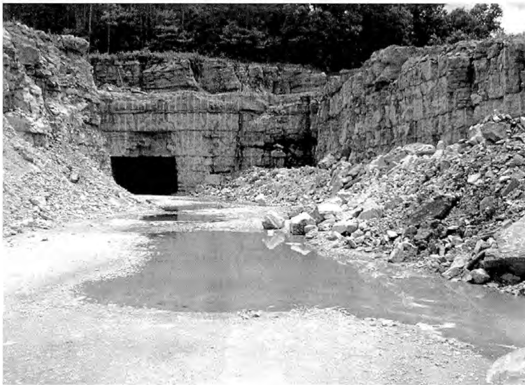
Figure 24. North entrance of the mine below Ky. 421.
