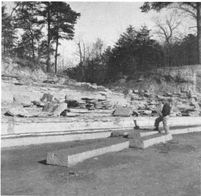
Fig. 27. Sandstone quarry located on Kentucky Highway 927, about 3 miles southwest of Parkers Lake, McCreary County. The stone is removed in slabs ranging in thickness from 3 to 8 inches. Minute shale partings between the layers of sandstone facilitates quarrying. Stone from this quarry has been used for construction at duPont Lodge, Cumberland River bridge, and schoolhouses at Monticello, Whitley City, Parkers Lake, Pine Knot, and other communities. It is thought to be lower Breathitt in age, and thus lies above the layers forming the Falls.
