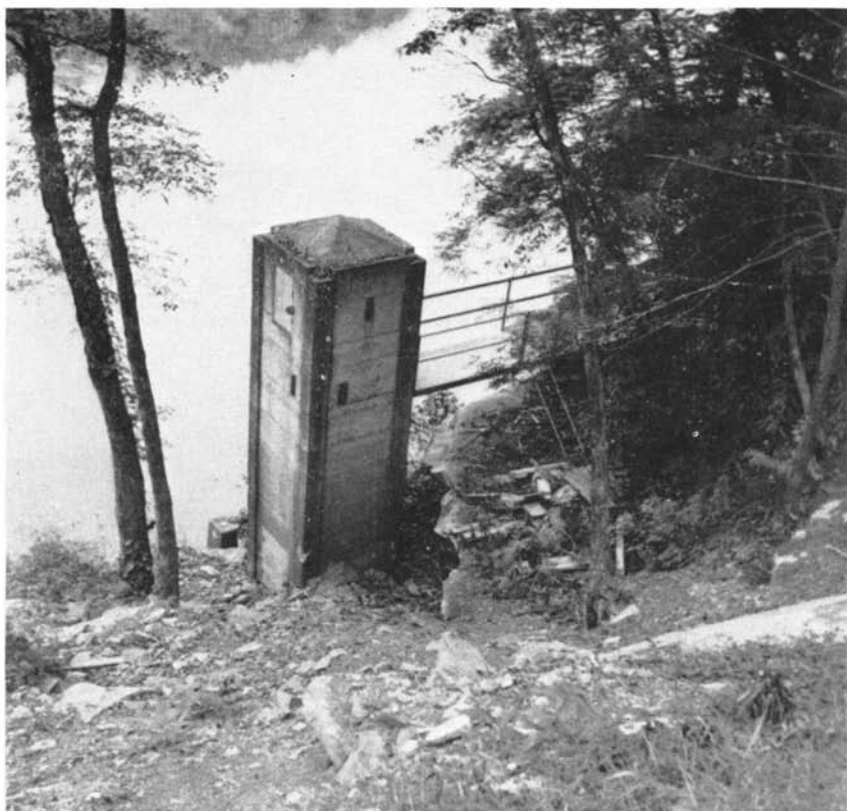
Fig. 15. Stream-gaging station on Cumberland River above Cumberland Falls. Records of the stream's behavior and characteristics are automatically gathered here. Knowledge of the variations in streamflow is desirable and important for practically any use of water or any water project. Published records for this point indicate variations in streamflow from a minimum of 8.5 cubic feet per second to a maximum of 59,600 cubic feet per second. This stream-gaging station is the oldest station now in operation in Kentucky.
