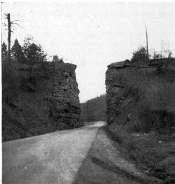
Fig. 12. Road cut through top 54 feet of sandstone at the top of the Lee formation one-fourth mile north of Staffordsville on Kentucky Route 172.
