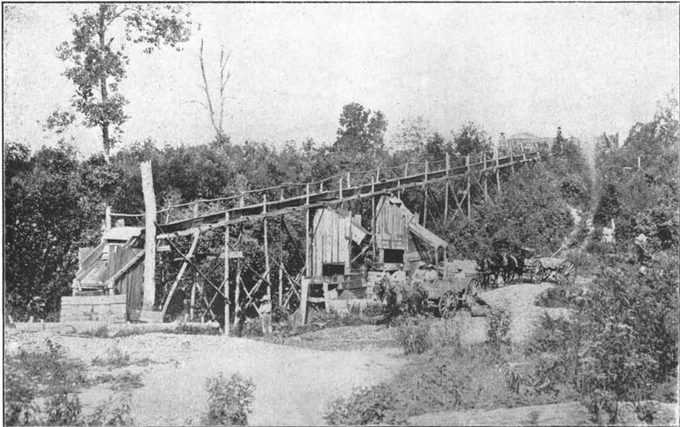
GRAVITY TROUGH WASHER AT TABB MINE.
