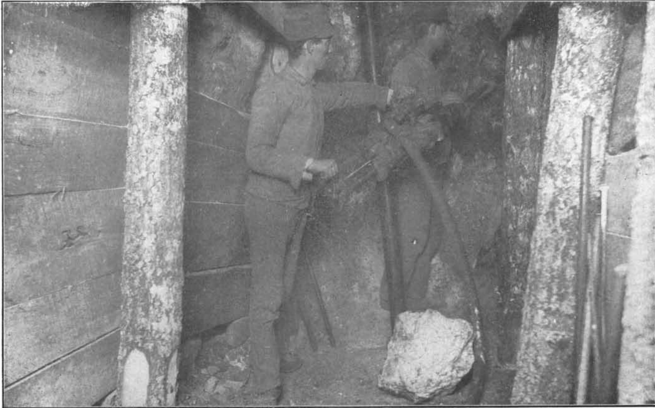
Riley Mine: Drifting at 35 Feet Level. Shows 4 Feet Vein of Galena-bearing Fluorspar; also method of timbering.
