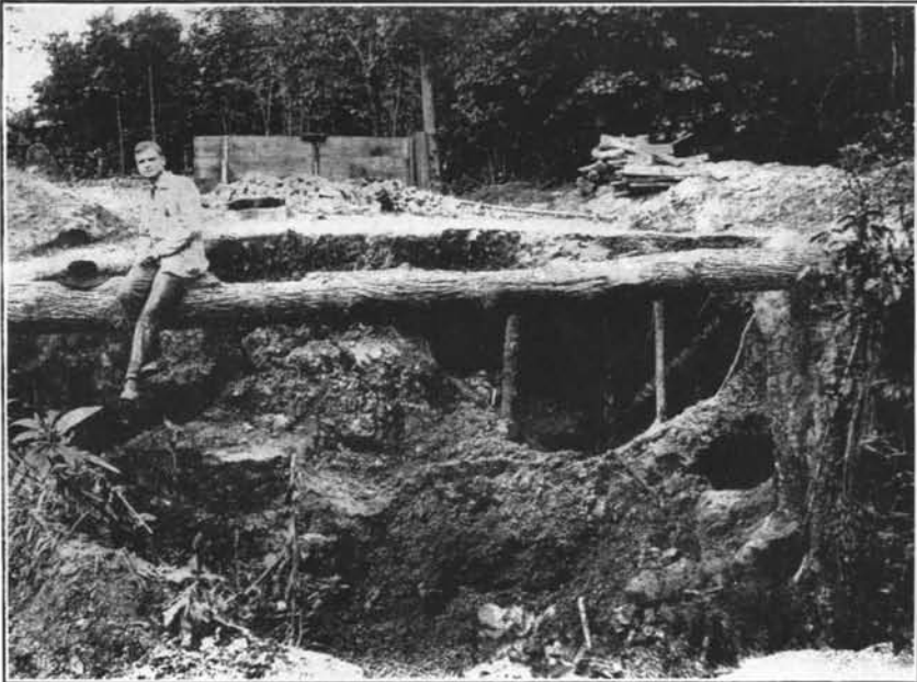
REED GRAVEL FLUORSPAR PIT. Drifting Just Below Grass Roots.
