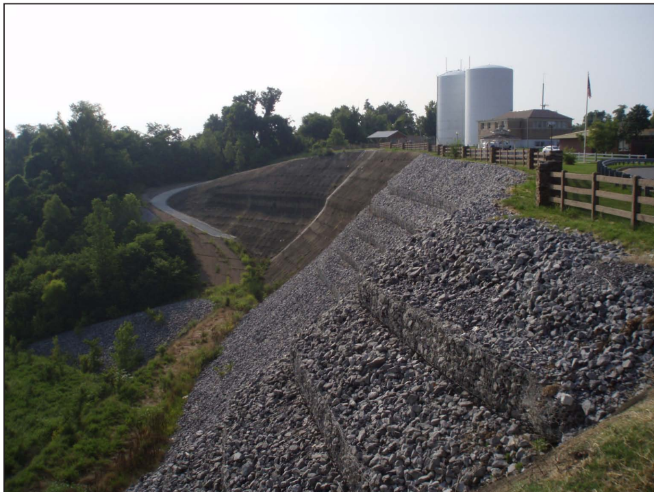
Figure 2. Repaired landslide in Hickman, Fulton County.
