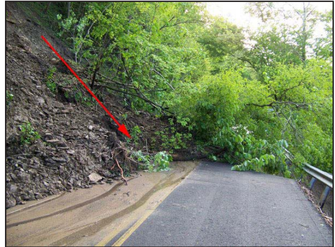
Figure 4. Left: The driving and resisting forces on a slope. W is the weight of the block. Right: A landslide along Big Eddy Road, Franklin County. This slide resulted from excess rainfall that increased the pore-water pressure, which decreased the strength of the material. The steep slope and clay-rich rocks were the underlying causes.
