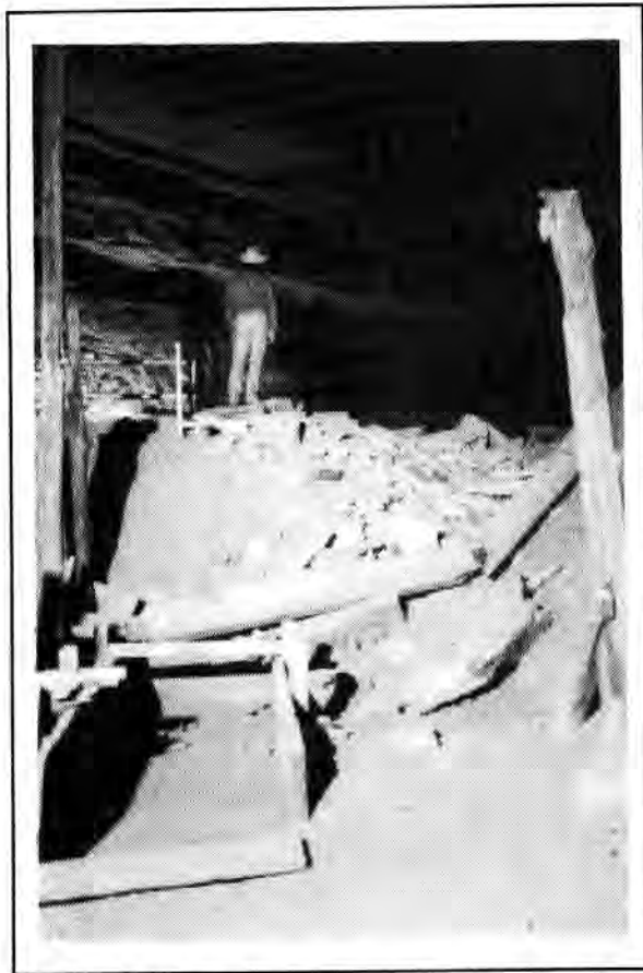
Figure 16. Damage to saltpeter mining artifacts from a large rockfall in January of 1994.
