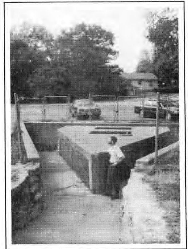
Figure 28. Specially designed trash rack protecting a drainage well in the parking lot of the Glendale Baptist Church (Stop 3).
