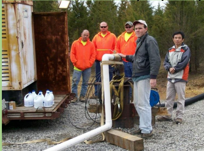
Assisted with pump set up
