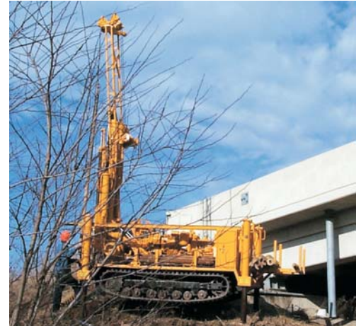
▲ Kentucky's Transportation Cabinet regularly repairs structures, such as this overpass, that are damaged by geologic hazards, including landslides and sinkholes.
