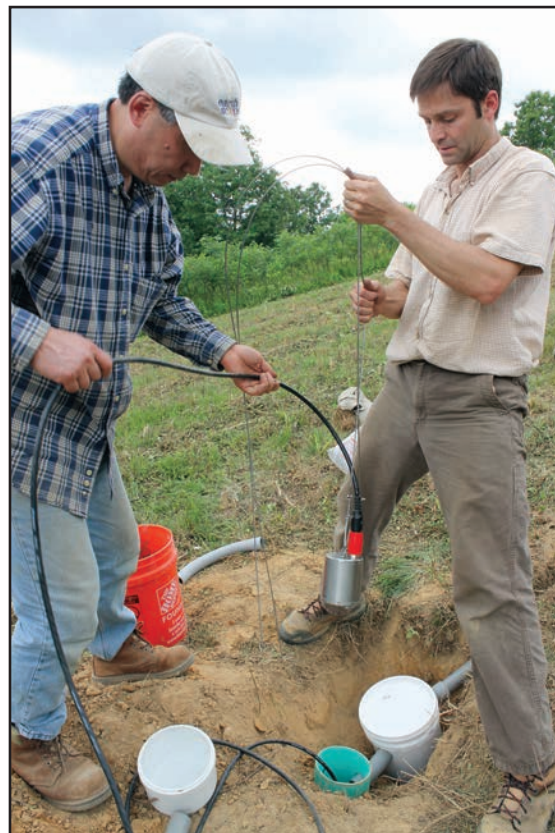
Zhenming Wang and Seth Carpenter install a new seismometer as part of the temporary monitoring network in eastern Kentucky.
