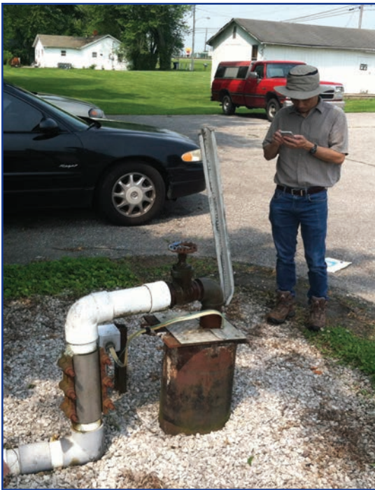
Junfeng Zhu collects GPS location coordinates during an inspection of a water-supply well in Elizabethtown.
