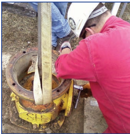
Glynn Beck prepares to remove a turbine pump collar prior to conducting a borehole video inspection of an irrigation well at the Murray State University Agricultural Farm in Murray.
