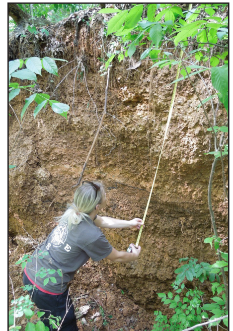
Amy King measures a scarp at the landslide near the closed Ledbetter Bridge.
