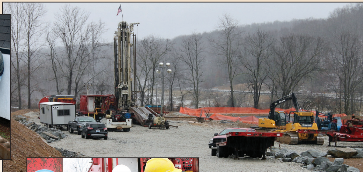
A drilling rig is set up on the Hanson Aggregates property in Carter County for the eastern Kentucky deep storage test project.
