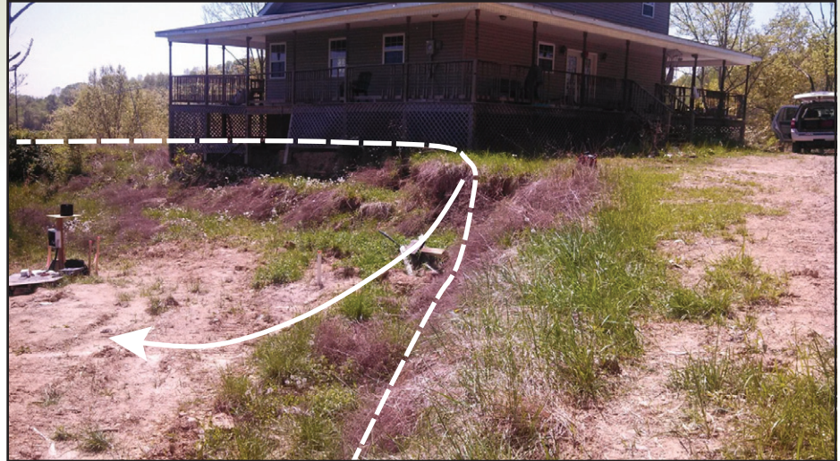
Meadowview landslide research site. The main scarp is outlined with a dashed line and the arrow shows direction of movement. The rain gage station is visible at left.
