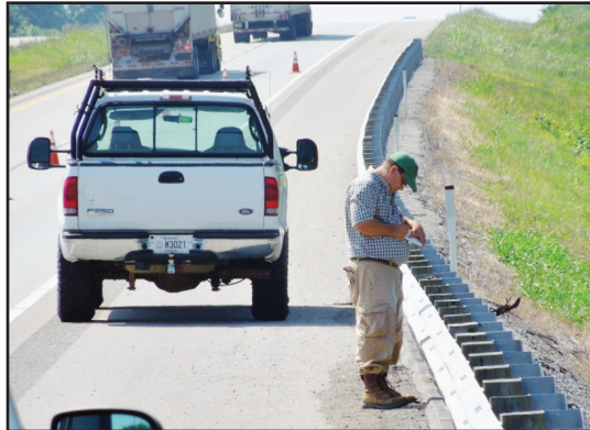
Scott Waninger gathered information on a road-fill failure along the Natcher Parkway in Ohio County.
