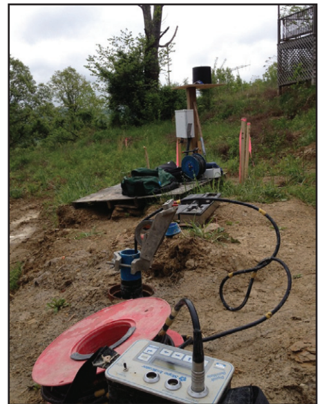
Monitoring instrumentation used for data collection at the landslide site. Inclinometer and data logger shown in the foreground and rain gage and water level transducer box shown in background.
