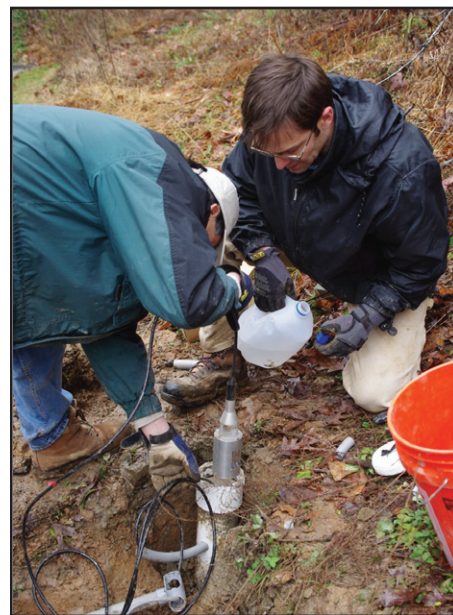
Zhenming Wang and Seth Carpenter install the new seismic station behind the Perry County Public Library.
