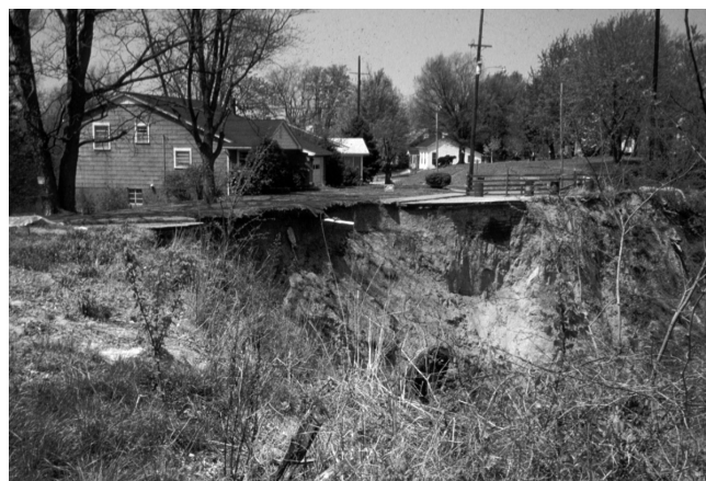
Landslides, like this one on Magnolia Street in Hickman, Ky., threaten property. Photo by John Kiefer.
